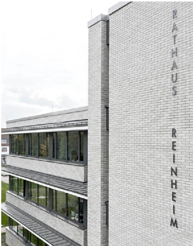
Living masonry made from Röben ceramic brick slips.
