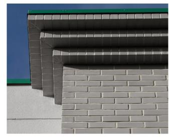
2. The insulation and reinforcement layer remain consistently thick, and the brick slips are applied in different thicknesses (14 mm / 25 mm). A detailed examination is required in this case.
