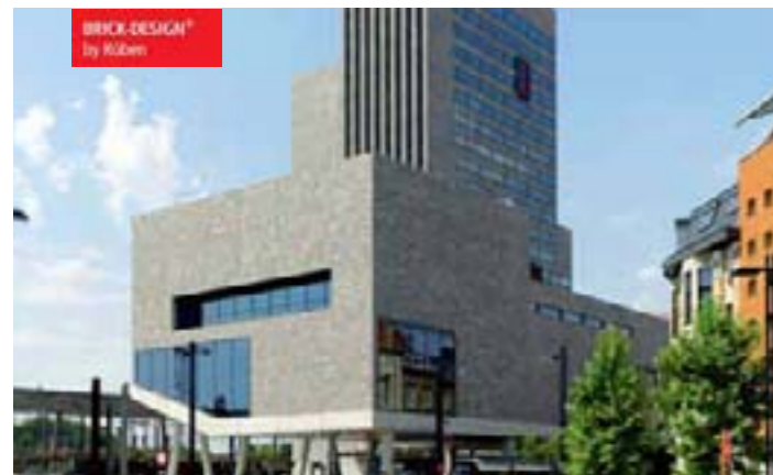
BRICK-DESIGN® by RÖBEN Building Office complex in Gent (B) Architects PoPONCINI Lootens, Antwerp (B) Facade Röben ceramic clinker bricks, YUKON, granite, BRICK-DESIGN® special assortment EXEMPLUM N°22
