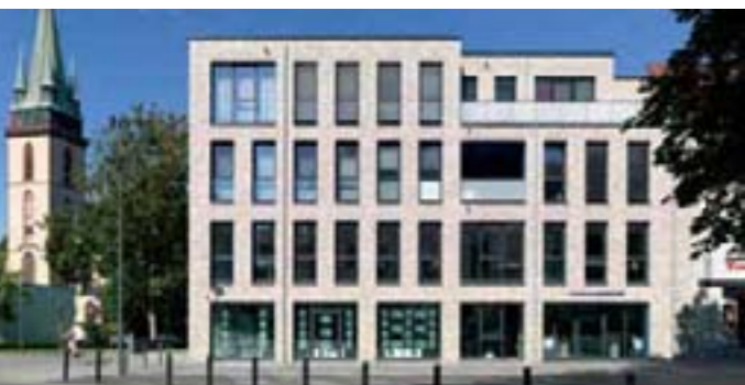
Powerful end point - Residential and commercial building in Lünen, page 24
