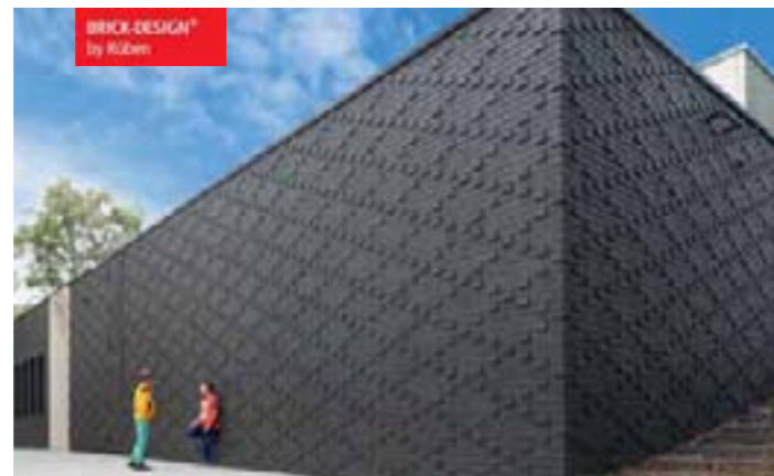
BRICK-DESIGN® by RÖBEN Building School canteen in Frankfurt/Main Architects dirschl.federle_architekten Facade Röben clinker bricks, FARO, black-nuanced, smooth BRICK-DESIGN® EXEMPLUM N°22
